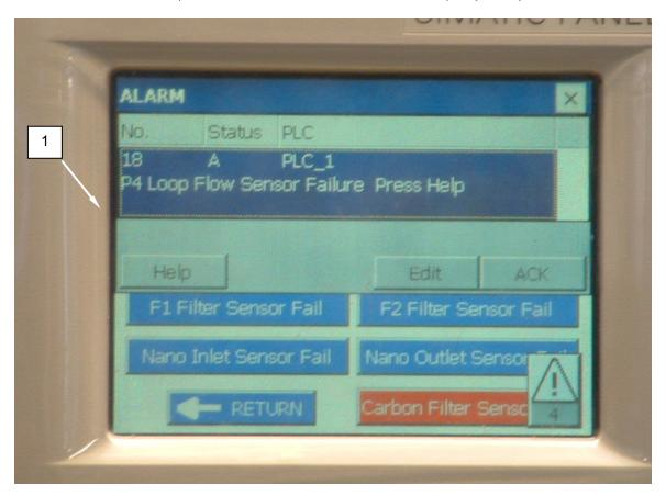
Figure 16. P4 Loop Flow Sensor Failure Alarm on PLC Display.
