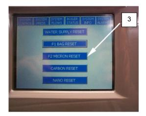
Figure 24. Resetting System Alarms.
