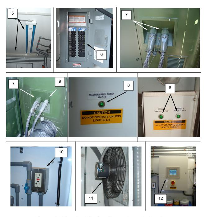
Figure 3. Lighting, Circuit Breakers, Receptacles, and Exhaust Fan.
