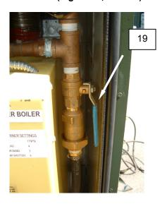
Figure 14. Boiler Water Inlet Drain Valve (V-38).
