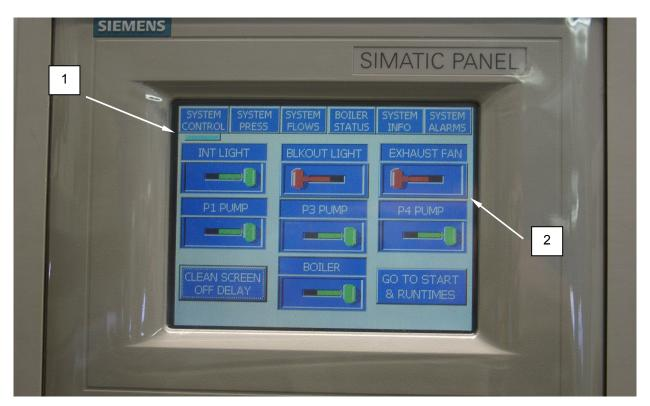
Figure 5. Operate the Exhaust Fans.
