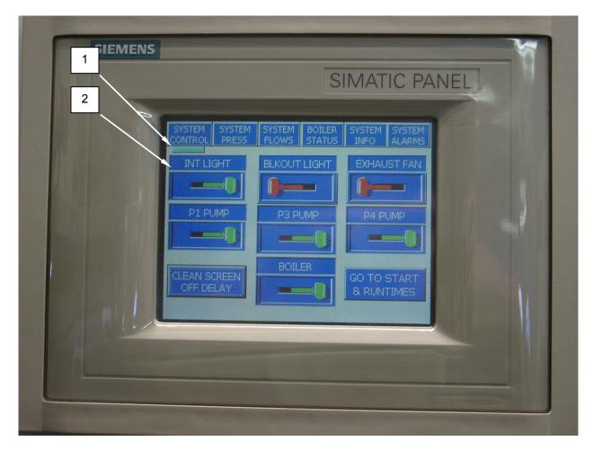
Figure 3. Operate the Interior Lighting.
