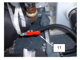
Figure 8. P-3 Pump Drain Valve.
