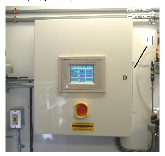
Figure 1. PLC Control Panel.
