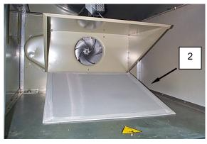
Figure 2. Replace the Dryer Lint Screen.
