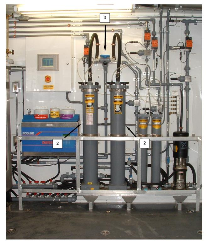
Figure 7. F1 Bag Filter is Clogged – P3 Pump is Stopped Alarm on PLC Display.
