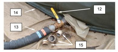
Figure 12. Prepare the 3000 Graywater Tank for Movement.
