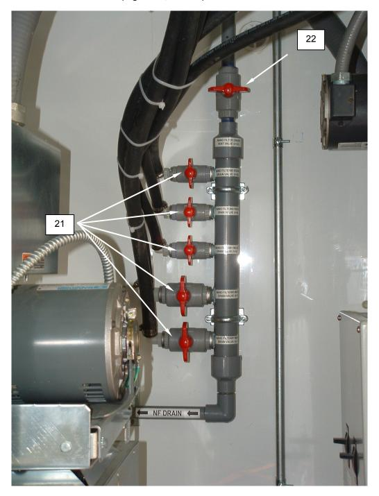
Figure 13. Vent Valves and Nanofilter Drains.
