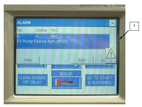
Figure 22. P3 Pump Alarm on PLC Display.
