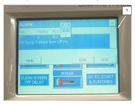
Figure 24. P4 Pump Alarm on PLC Display.
