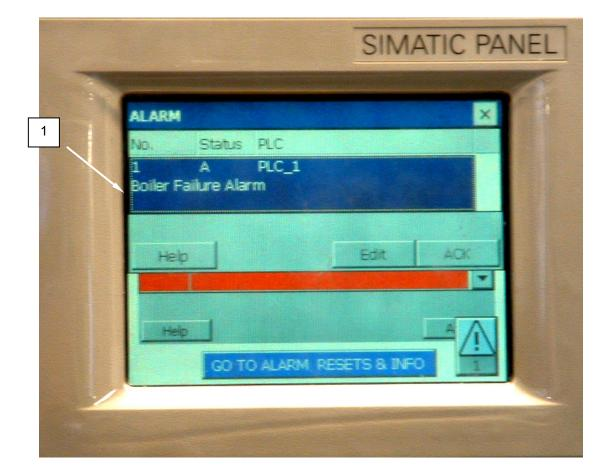
Figure 3. Boiler Failure Alarm on PLC Display.
