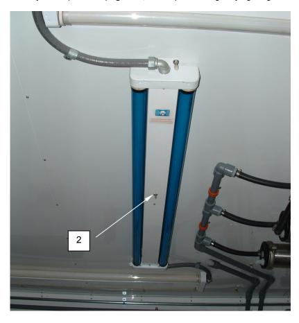
Figure 2. Switch ON the Battery Backup for Emergency Lighting.
