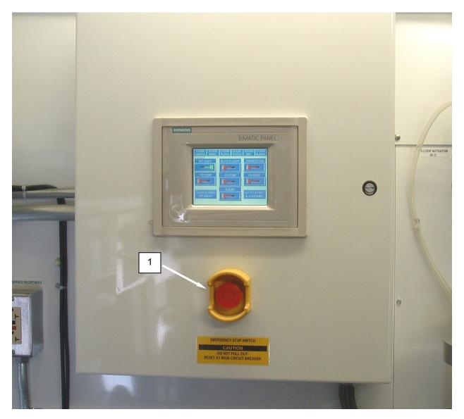
Figure 1. Emergency Shutdown Switch.
