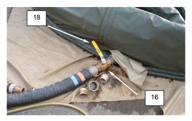
Figure 6. Install the Valve Handle on the 3000-Gallon Water Tank.
