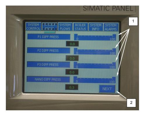
Figure 14. System Press Display.
