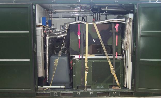
Figure 33. Securing the Components with Straps.
