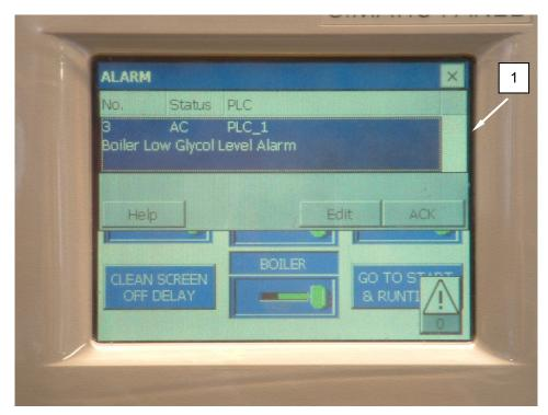
Figure 9. Boiler Low Glycol Alarm on PLC Display.
