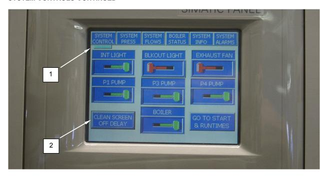
Figure 8. Operate the Clean Screen off Delay.
