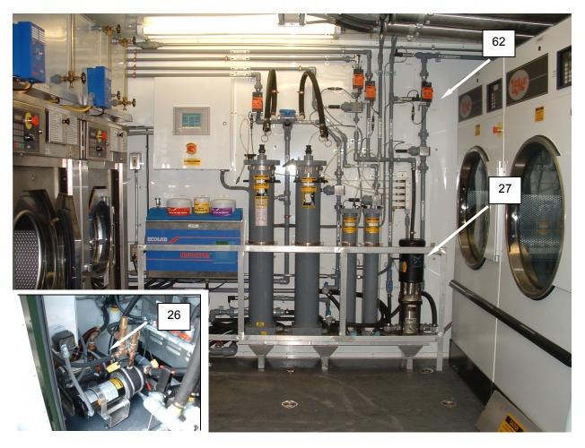
Figure 24. Weekly PMCS – Water Treatment System.
