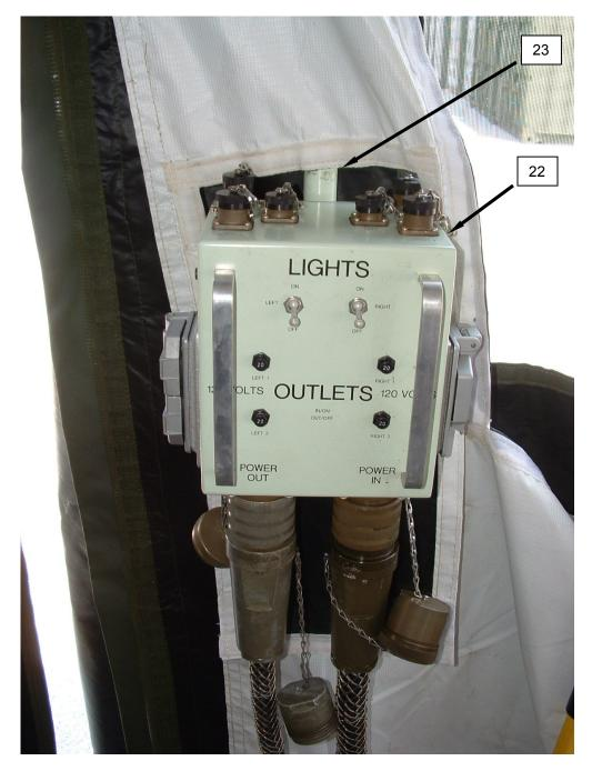
Figure 27. Remove Distribution Box and Stand during NBC Imminent or Actual Attack.
