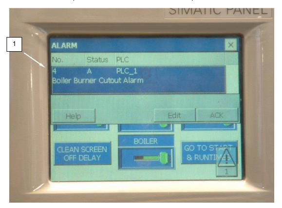
Figure 28. Boiler Burner Cutout Alarm on PLC Display.
