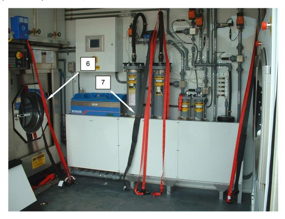
Figure 6. Attach Straps to D-Rings.
