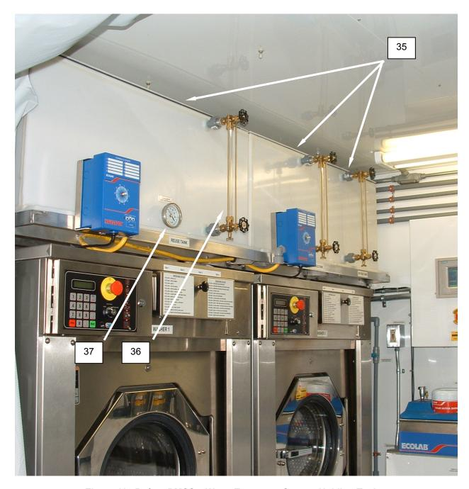
Figure 12. Before PMCS – Water Treatment System Holding Tanks.
