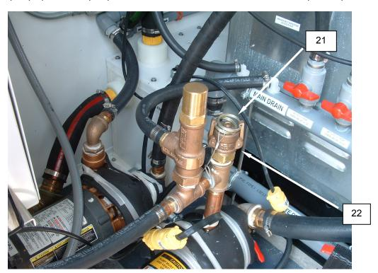
Figure 16. P-1 Pump Priming Standpipe.
