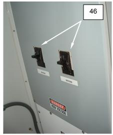
Figure 13. Check Dryer Phase Indicators.
