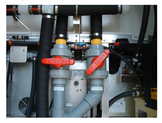
Figure 5. Valve Setting for Minimum Water Reuse.
