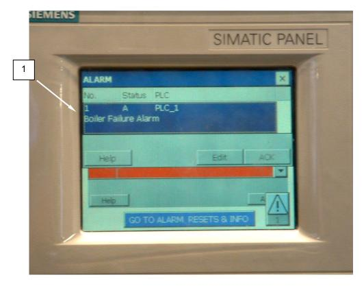
Figure 26. Boiler Failure Alarm on PLC Display.
