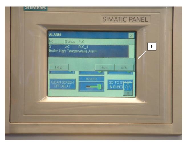
Figure 7. Boiler High Temperature Alarm on PLC Display.
