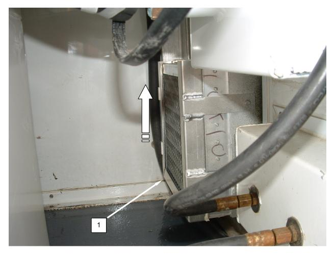
Figure 4. Replace the Boiler Air Filter.
