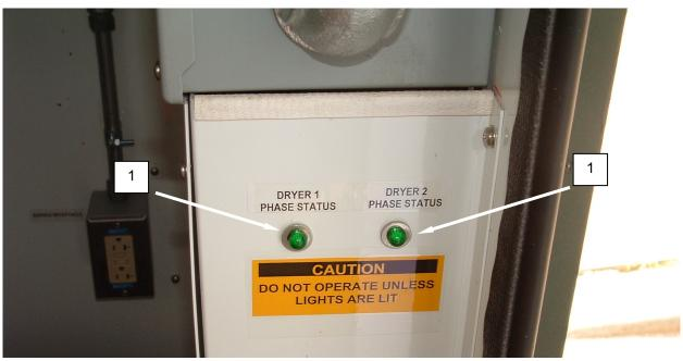
Figure 1. Phase Sequence Indicator Lights.
