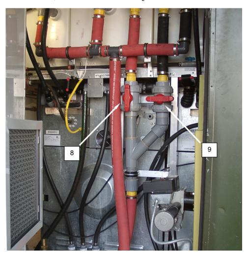
Figure 3. Valves V-15 and V-16.
