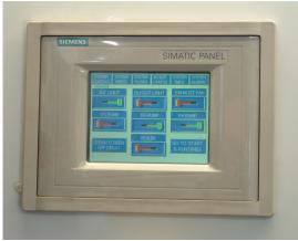
Figure 10. Boiler Low Glycol Alarm on PLC Display.
