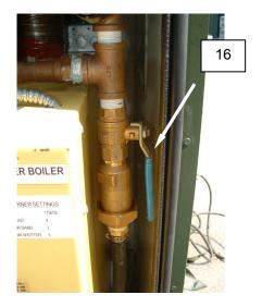
Figure 10. Boiler Water Inlet Drain Valve.
