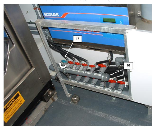
Figure 12. Location of Drain Manifolds.
