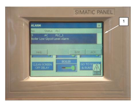
Figure 31. Boiler Low Glycol Alarm on PLC Display.
