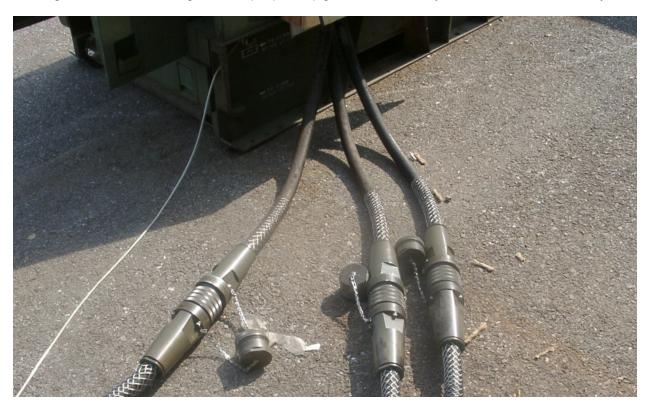
Figure 10. Connect 100 A Pigtail Cables to Generator.
